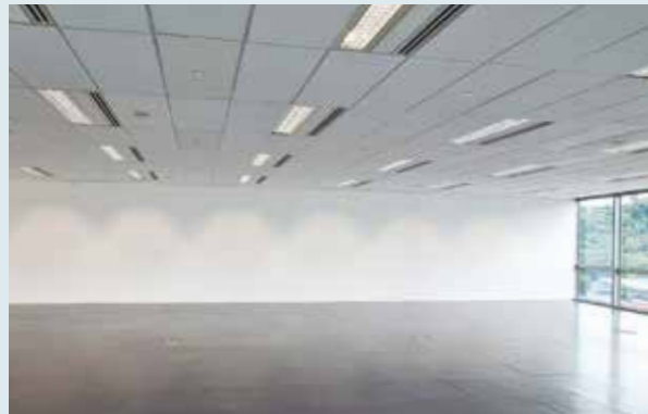
Implemented circularity principles by retrofitting light fixtures at MBC and BOAHF with LED tubes while reusing the rest of the lighting fixtures
